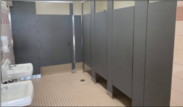
Typical Student Restroom
