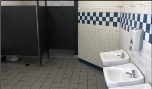
Typical Student Restroom
