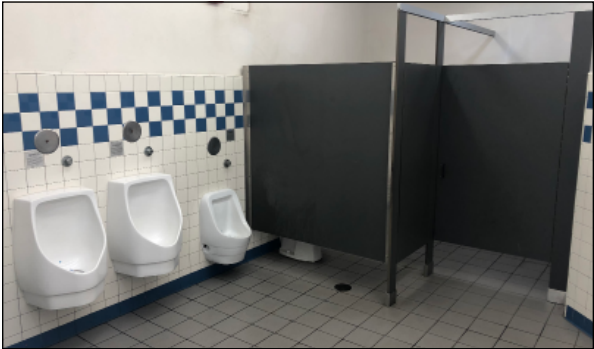
Typical Student Restroom
