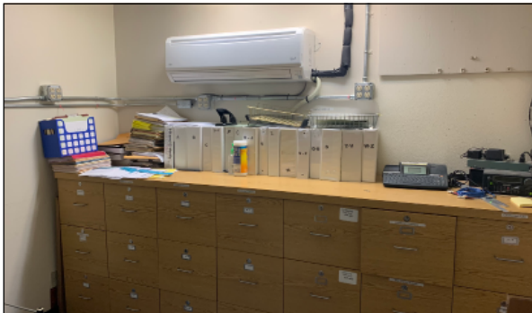
Office Interior - Administrative Services File Room
