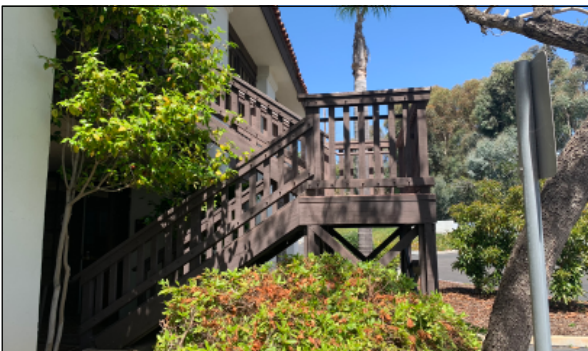
Office Exterior Stairwell
