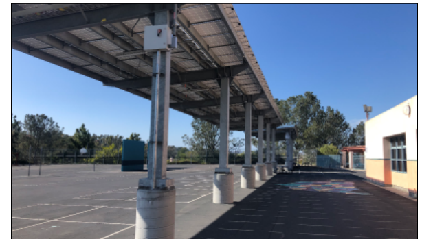
Solar Shade Structure and Hardcourts
