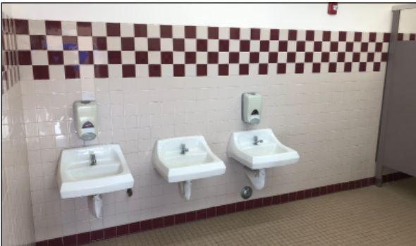
Typical Student Restroom
