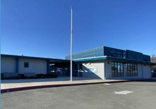
San Miguel / Juntos Elementary School 777 San Miguel Ave.
